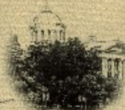
Anderson County Courthouse
